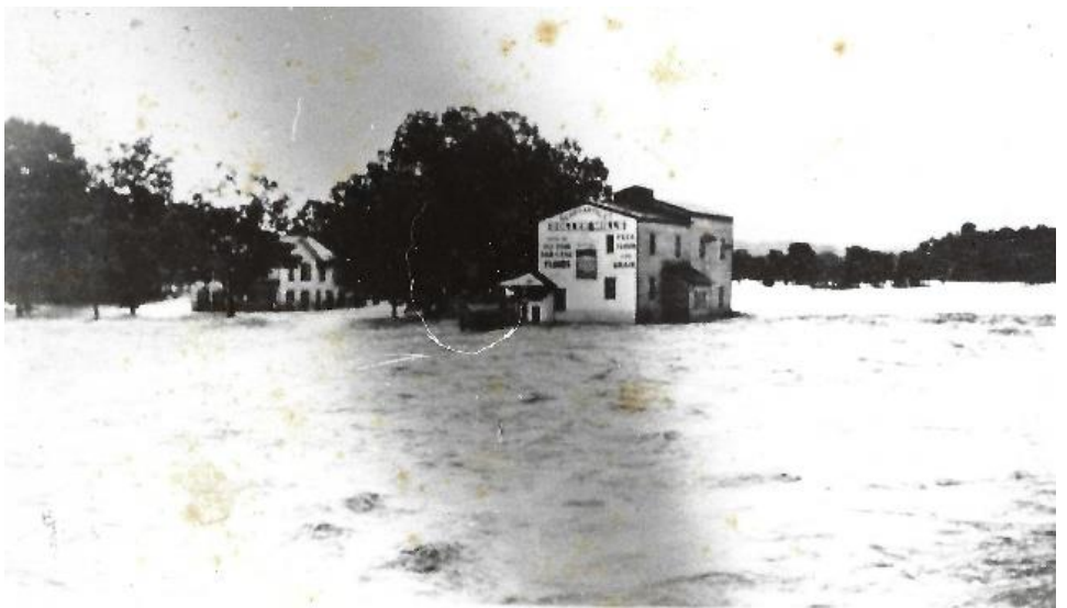
Hansmann's Mills mid-flood July 1935
